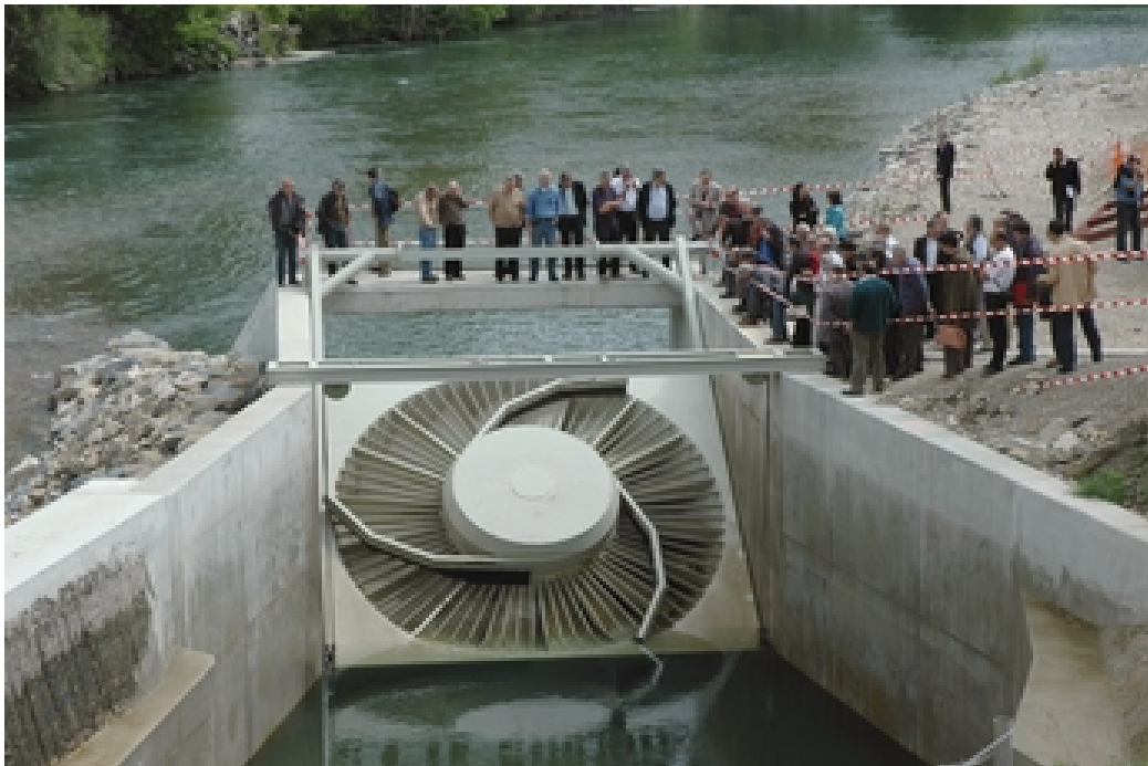
Figure 4.1. The MJ2 turbine at Millau
